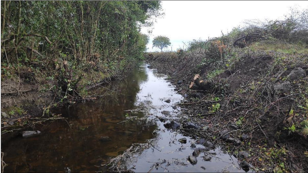
Plate 4.13 The historically straightened Clonmore Stream had been recently cleared of instream and riparian vegetation upstream of the survey site
